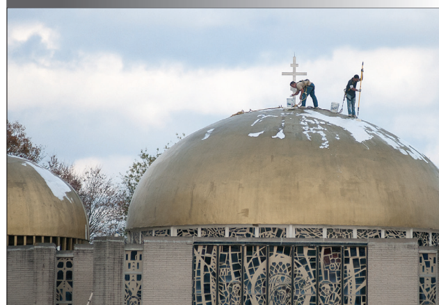
CHLOE ELMER / STAFF PHOTOGRAPHER Men work on the roof of Our Lady of Perpetual Help Byzantine Catholic Church in Bristol Township on Tuesday afternoon.
